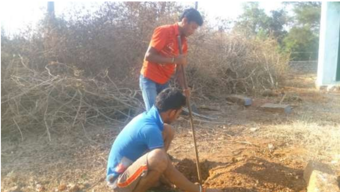
Fencing work by NSS Volunteers
