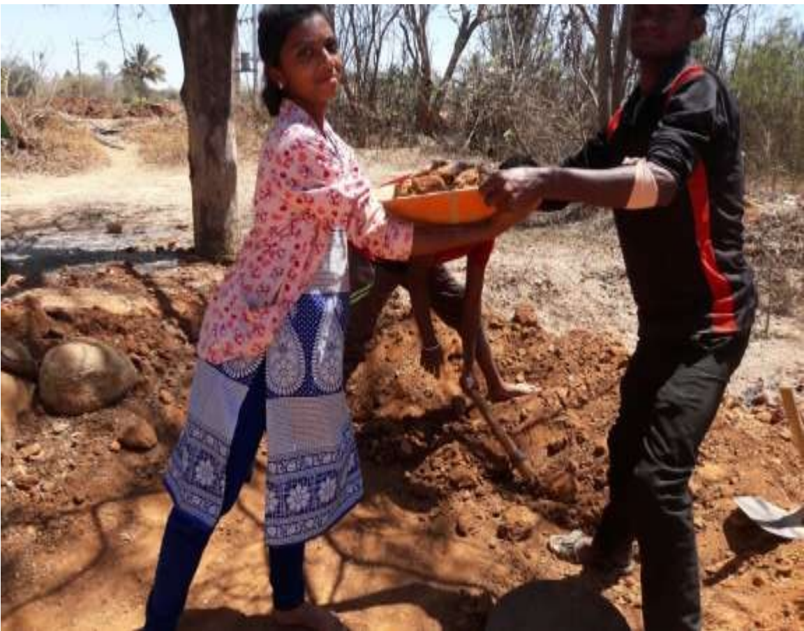
Construction Of Open Theater by Our NSS VOLunters
