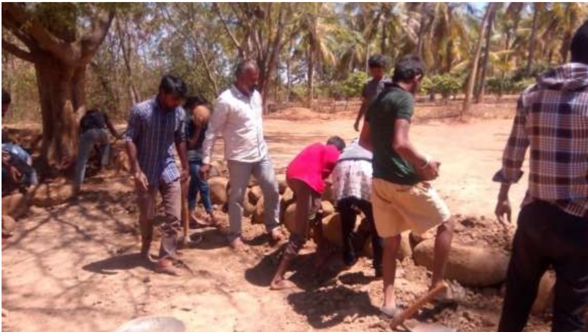
Open Theater Construction Work.
